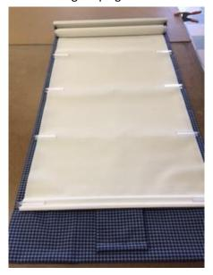
**6. Insert spring end of tube into bracket with adjuster wheel**. This bracket should be already screwed to your board.
