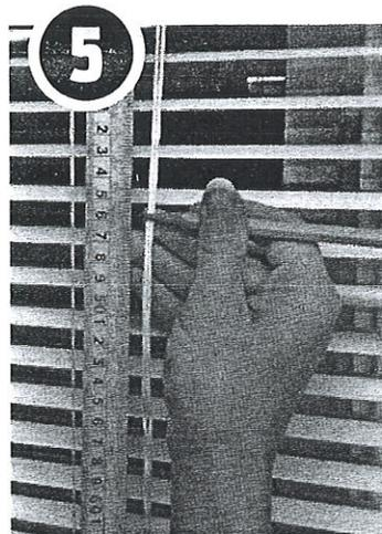
**5** With blind in the down position, measure from top of head rail down 14 inches, mark cords with a pencil.
