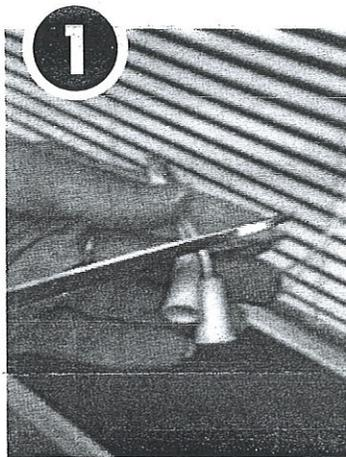
**1** With the blind in the down position, confirm fit of the Fashion Wand Head Rail clamp, then remove tassels with scissors and discard. Cut cord evenly, this will be your reference for keeping the blind level.
